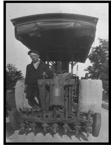
Tom Raish takes a photo break while working on Main Street. (year unknown)
